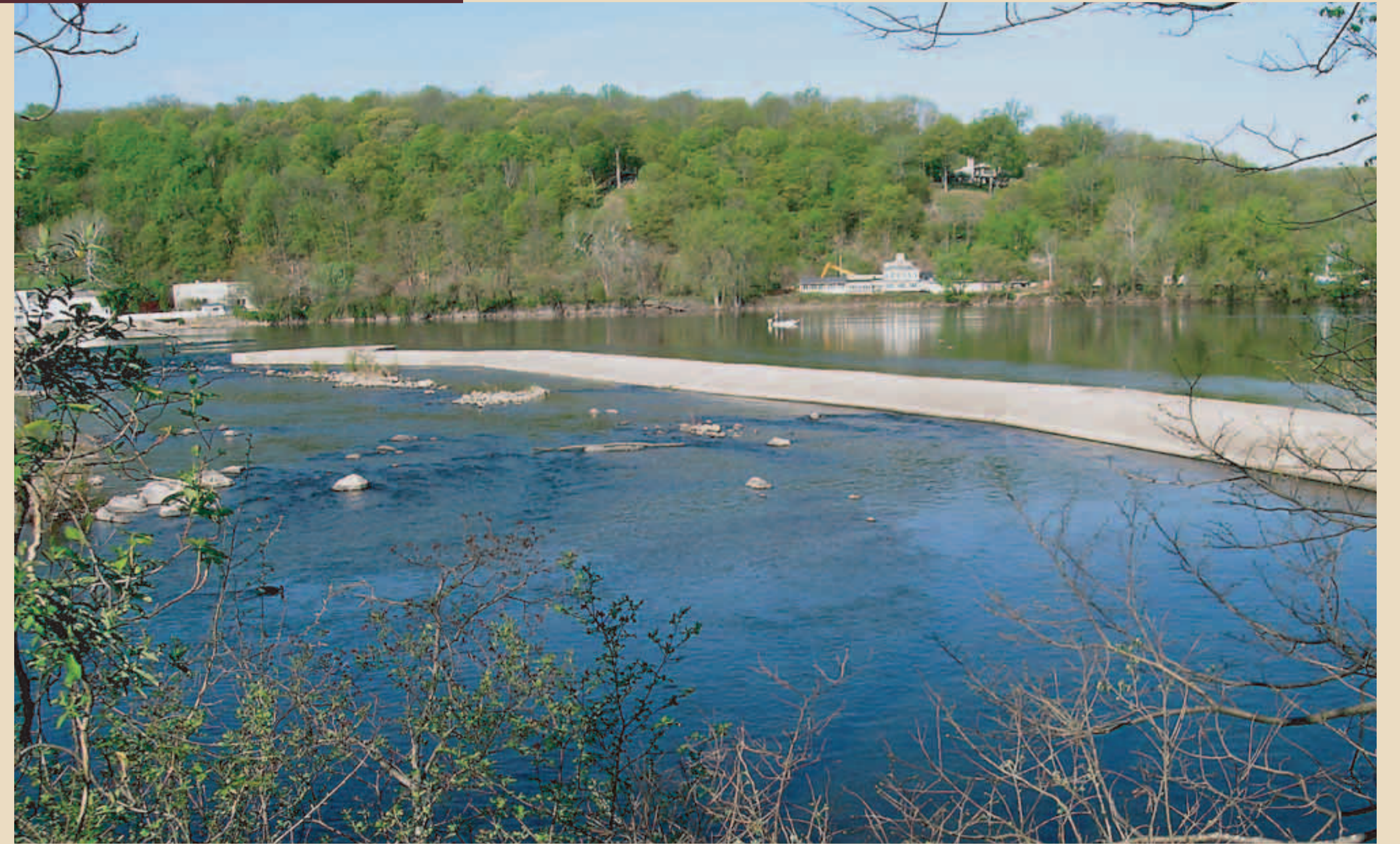
The wing dam at Wells Falls raised the river level so that water could be diverted into the canal.
