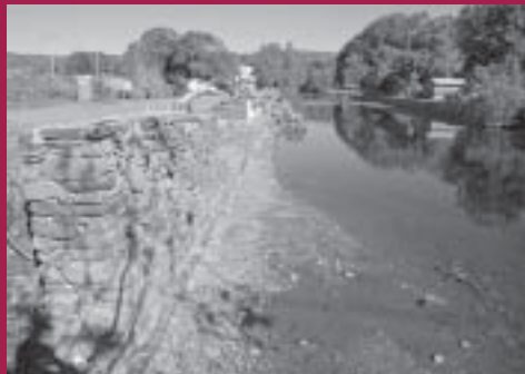
The 300-foot stone wall under construction at the Weissport Trailhead.
