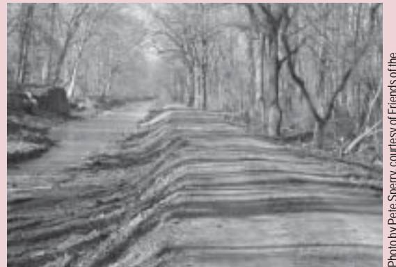
Repairs to the towpath near the David Library following September’s flood allowed the southern 25 miles of the Delaware Canal to be rewatered.
